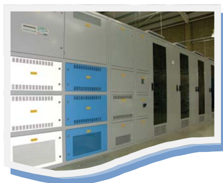
Composite construction arrangement STS—PDU.
