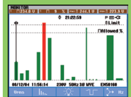
The System-Monitor overview screen gives instant insight into whether the voltage, harmonics, frequency, and the number of dips and swells fall outside the set limits.
