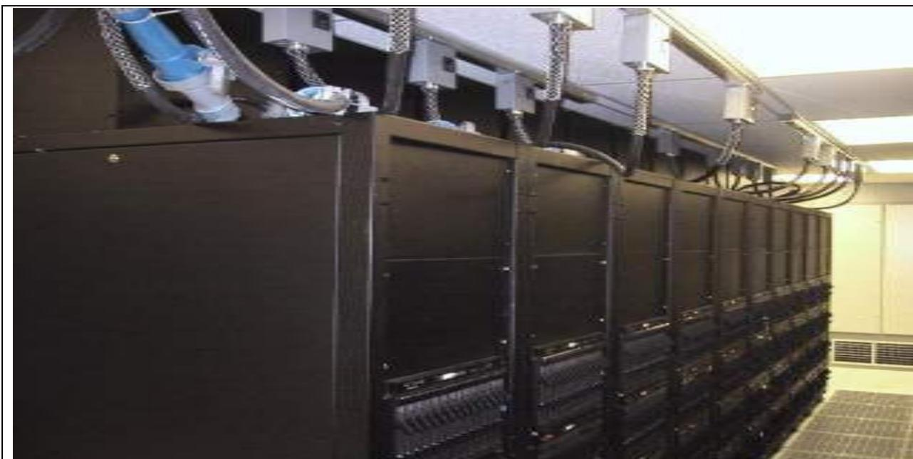
*Figure 3 : “Exotic” data center cooling technologies like this in-row liquid cooling system are costly to install and maintain. They also expose sensitive server hardware to the dangers of leaky pipes.*
